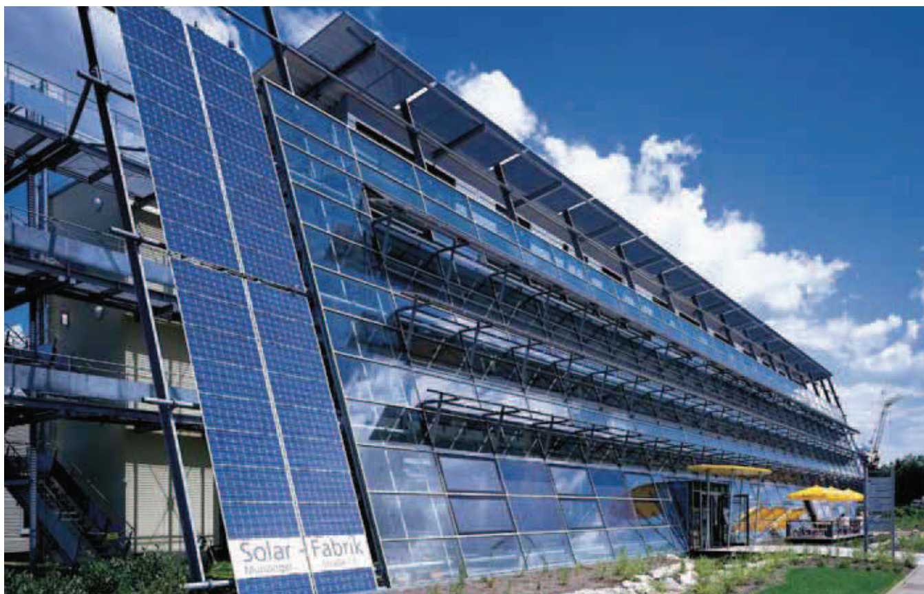
Ökowerk: The power required for module production is obtained by the Freiburg-based company Solar-Fabrik from cells on the façade and roof of its own factory. (Photo: Solar-Fabrik)
