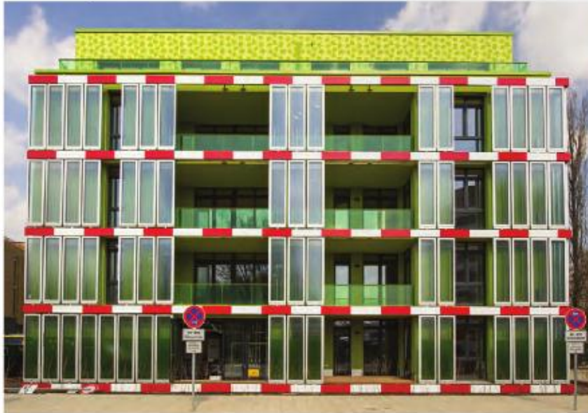
Algae house: In the façade of the "House with Bio Intelligent Quotient" in Hamburg algae use photosynthesis to produce heat for the apartments.
