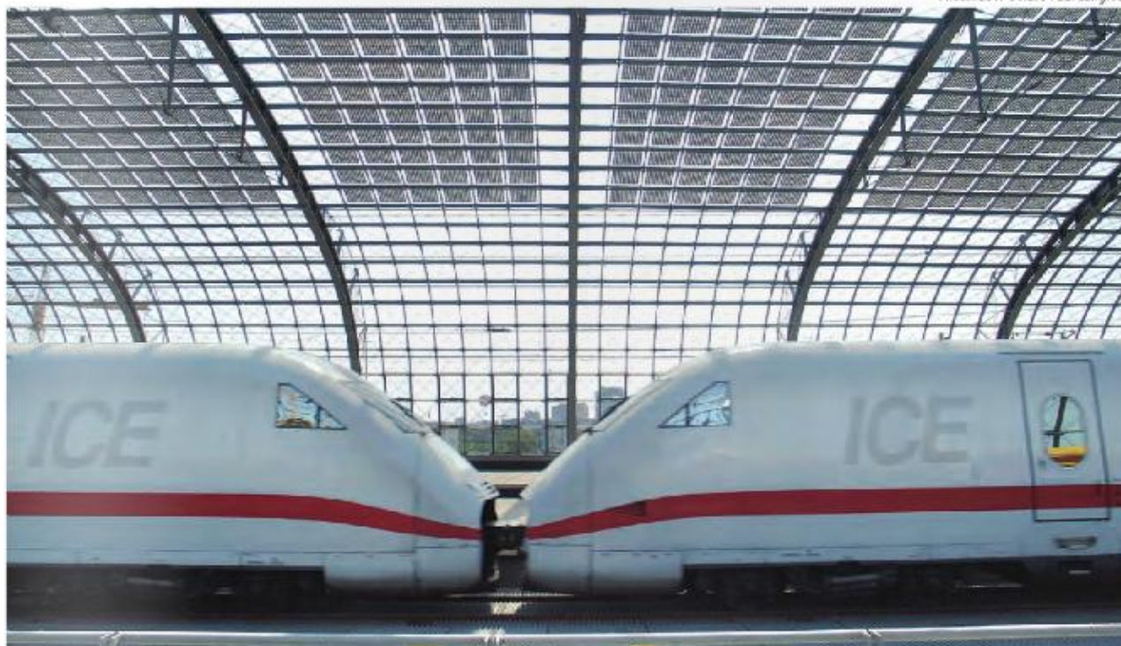
Field-tested showcase project: The roof of Berlin's main rail station clearly illustrates the advantages of BIPV: the modules generate electricity and at the same time transmit light.
