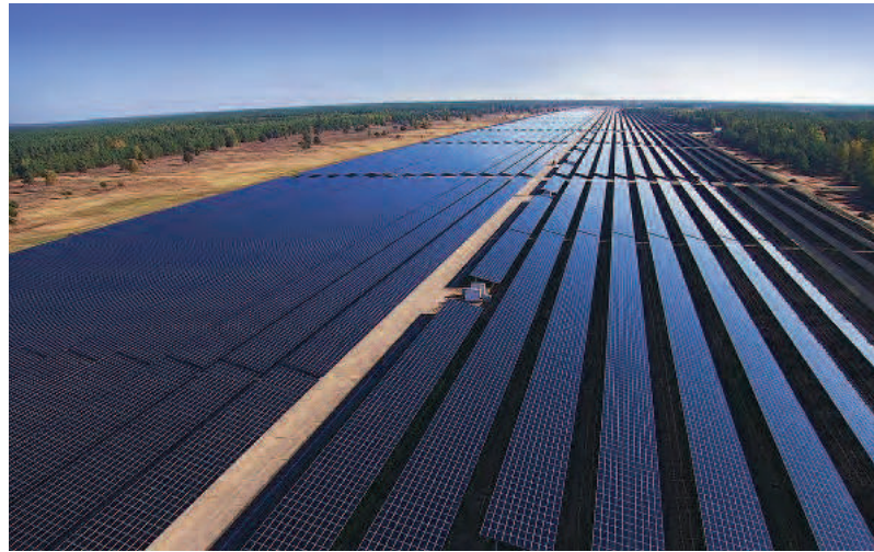
Thin-layer in rows: solar project developer Belectric has built Europe’s biggest photovoltaics power plant in Eastern Europe using cadmium-telluride modules by First Solar.
